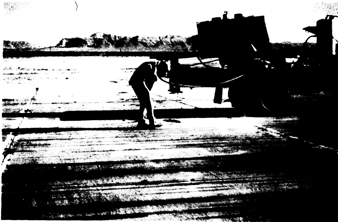
Figure 4-4. Sandblasting Equipment Cleaning Joints.
