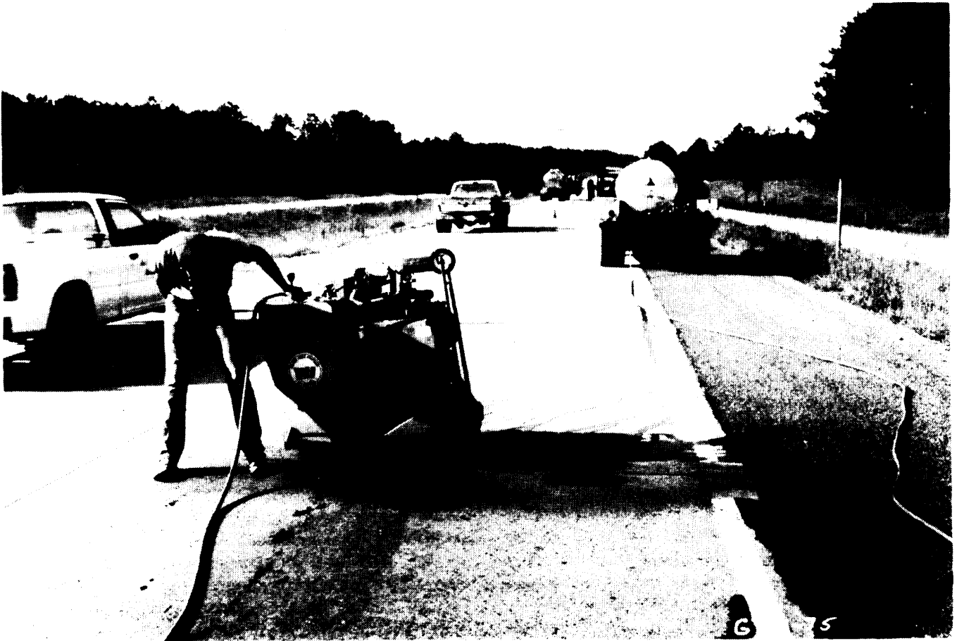
Figure 4-1. Concrete Saw Refacing Joint.
